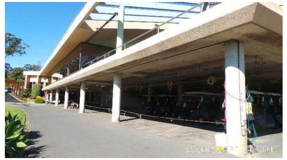
6. Undercover golf buggy storage area
