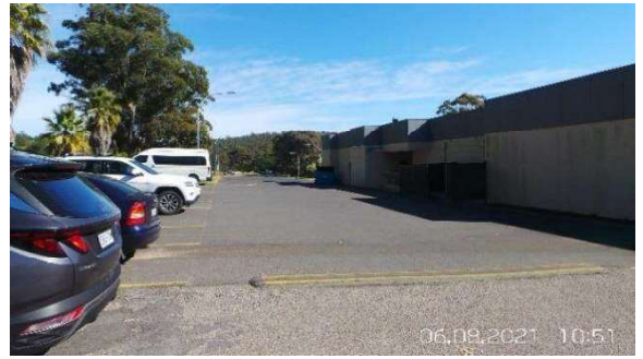
4. Southern elevation and adjacent car park
