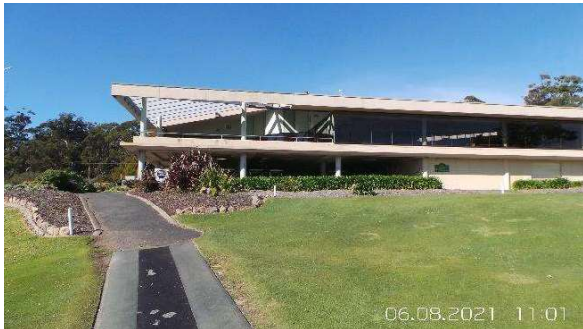
3. North-west elevation of clubhouse
